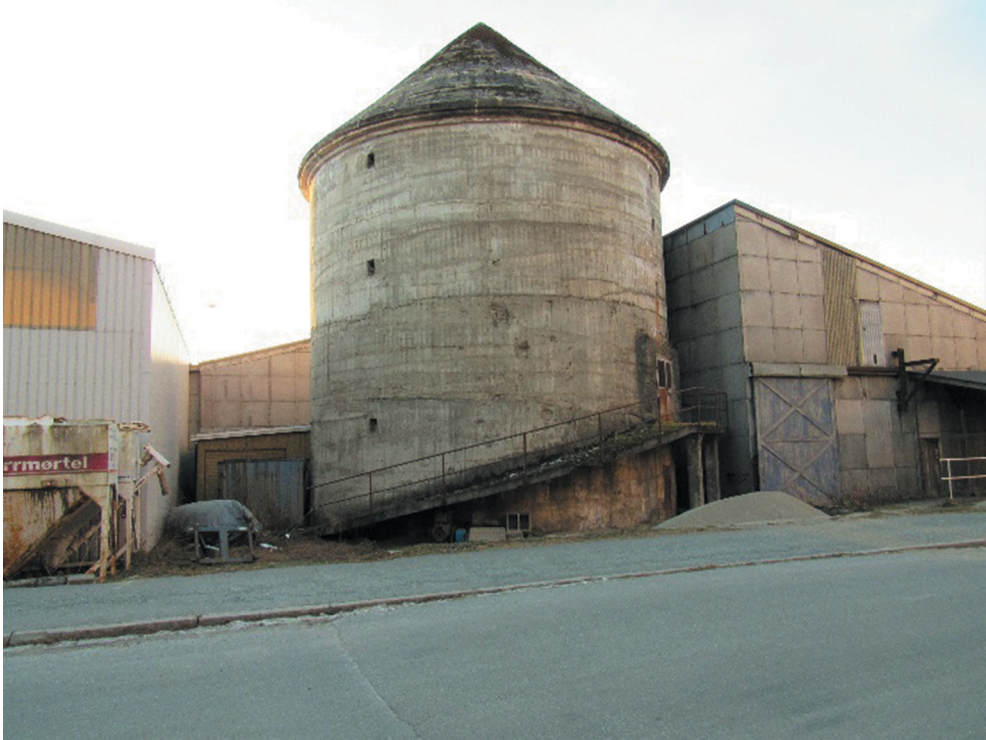
Figure 3: One of the pretty well-preserved air-raid shelters (Luftschutz Turm der Bauart Zombeck) on Ladehammer quay.
