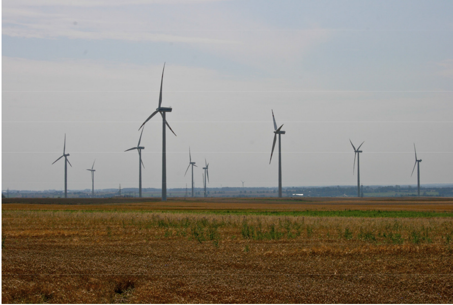
Figure 1: Wind farm near Lisewo, Poland, an example of almost regular matrix spacing. This type of spacing, being purely utilitarian and geometric, ignores unique properties of landscape.
