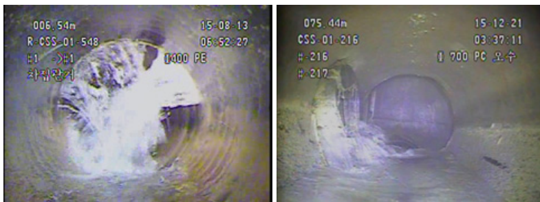
Figure 4: The pictures of internal interceptor sewer conditions in Seo-san.
