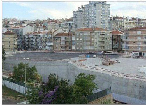
Figure 2: The CRIL during construction (Source: www.cril-segura.com ).
