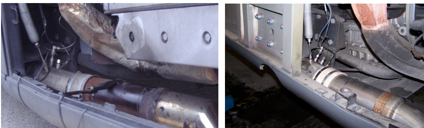
Figure 2: Exhaust gas flow meter with its Pitot tubes.
