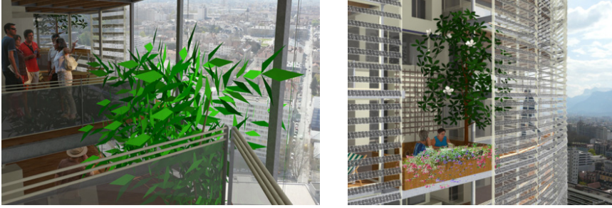
Figure 8: The Shell: the glass hull (left) and the photovoltaic shield (right).
