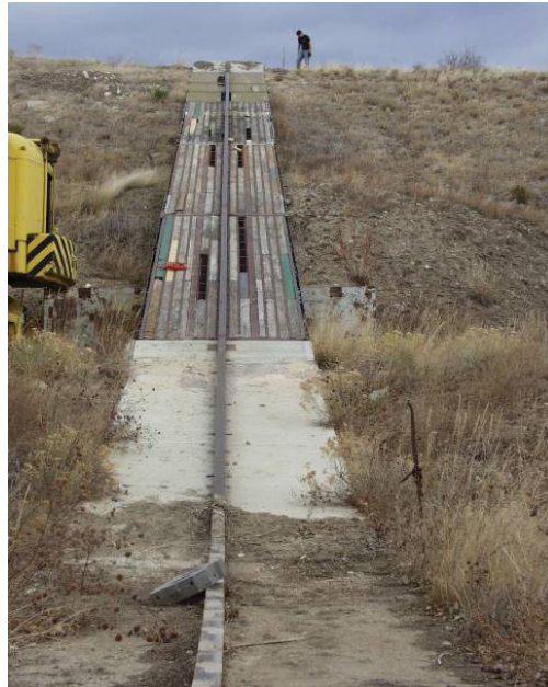
Figure 1: Current view of ramp.
