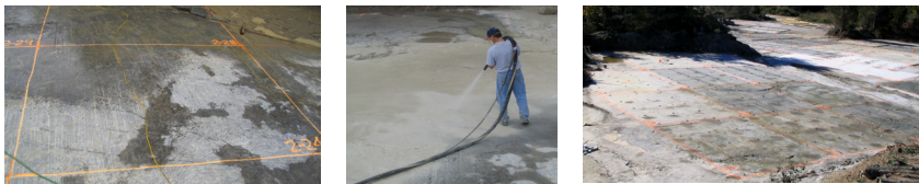
Figure 2: Views of cleared outcrop, TSL installation and prepared sites.
