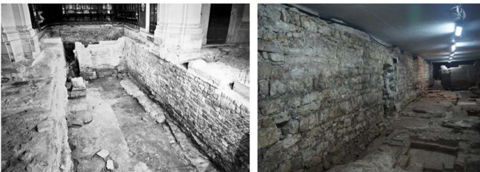
Figure 2: Photographs of the of the central nave underground during excavation and after finished floor slab. (Source: Institute for Restoration of Dubrovnik.)
