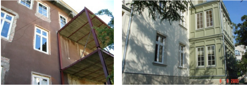
Figure 6: Veranda under construction (left) and veranda at present (right).
