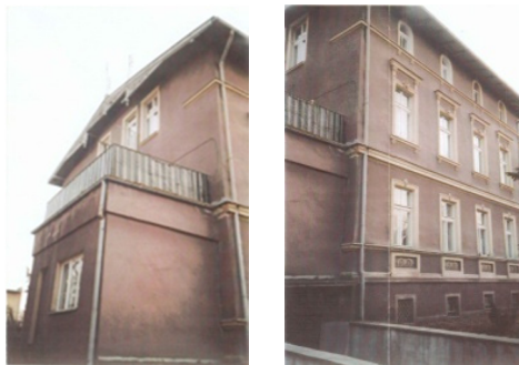
Figure 4: Façades before modernization with the brick lean-to.
