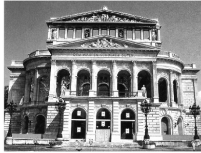
Figure 2: Old Opera in Frankfurt: substitution techniques erase war traces, damaging documentary value of matter in its appearance (picture: Brix [4]).
