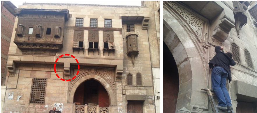
Figure 5: Façade of example 2.
