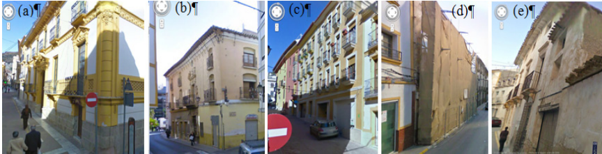
Figure 4: URM buildings before the earthquake (Google street view).
