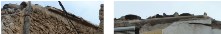
Figure 10: Masonry wall and timber ring beam.
