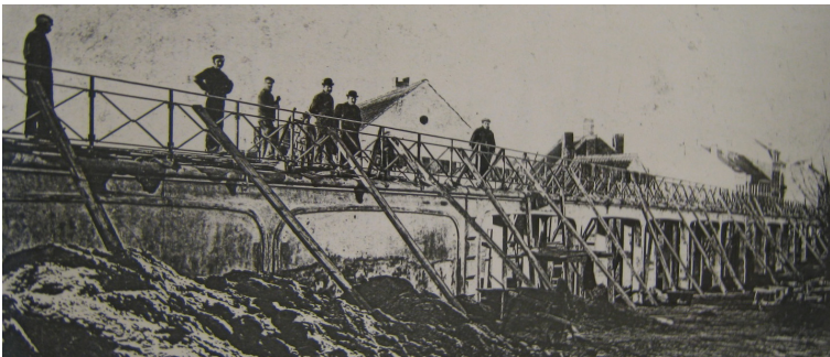
Figure 1: Colo-Hugues viaduct during construction in 1904–1905 [3].
