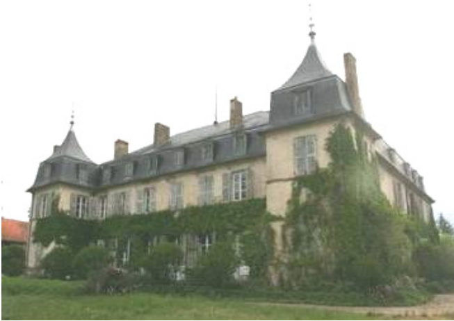
Figure 1: A chateau made of rammed-earth which was built about 300 years ago in France.
