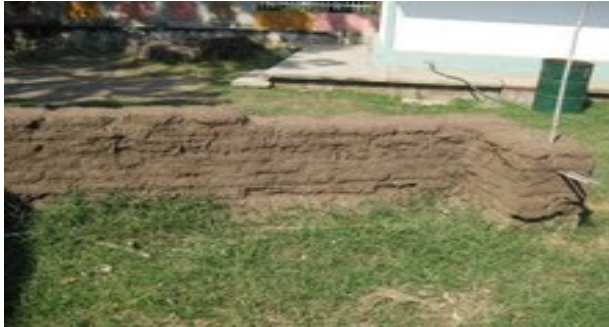
Figure 1: Building process of adobe wall. Picture: M. F. Elizondo (2009).
