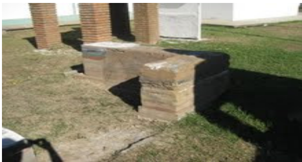
Figure 2: Experimental building with rammed earth wall. Picture: M. F. Elizondo (2009).
