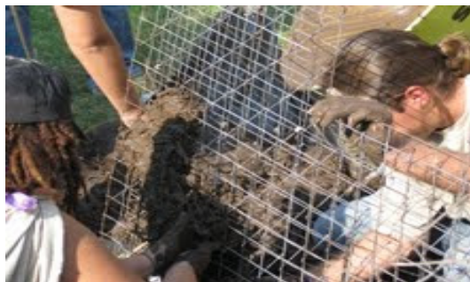
Figure 4: Architecture students building with techno-bajareque wall. Picture: M. F. Elizondo (2009).
