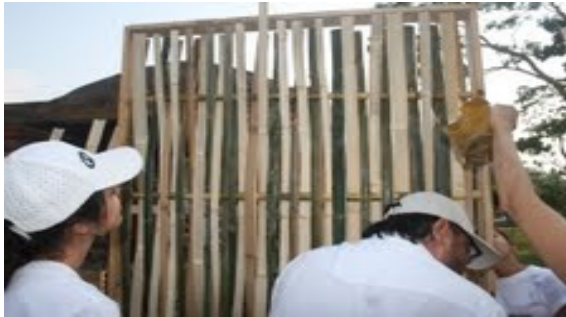
Figure 3: Building the vegetable structure of bajareque wall. Picture: M. F. Elizondo (2009).
