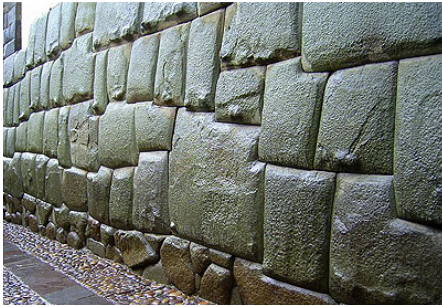
Figure 4: Heavily compacted dry-stacked stone masonry in Cuzco, Peru.
