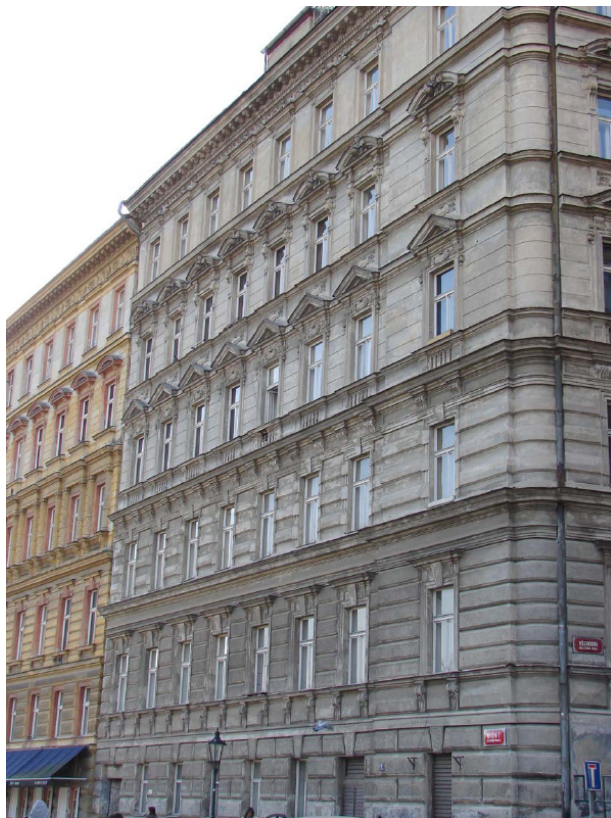
Figure 1: View of the assessed building.
