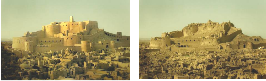
Figure 1: Bam before and after the earthquake.
