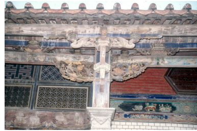
Figure 11: The architectonic expression of a traditional wood frame on the top of a column with classical order.
