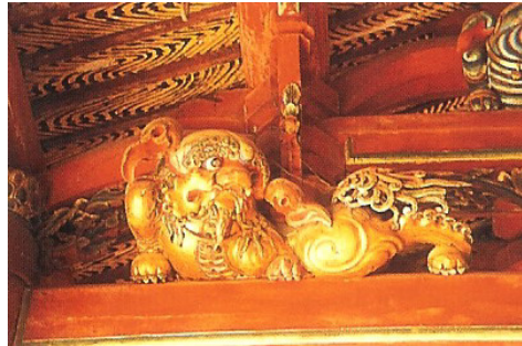
Figure 5: Decorated dragon of the column Figure 6: Lion-shaped wood block in a diedou structural frame.
