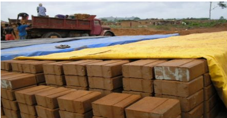
Figure 1: Interlocking blocks produced from laterite and used in Obasanjo low-cost housing estate, Ado-Ekiti, Nigeria.
