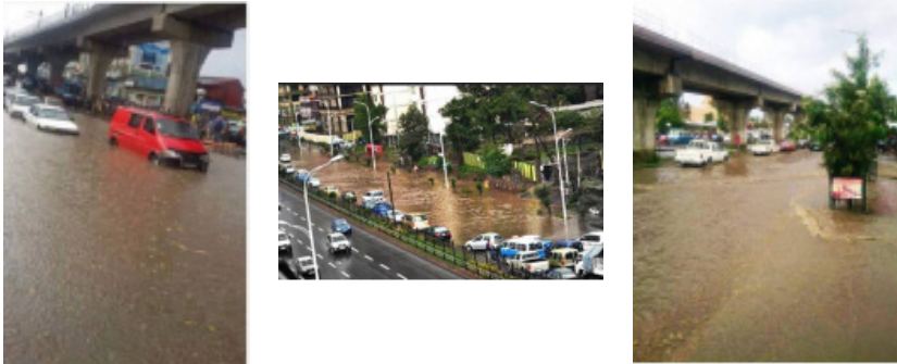
Figure 2: Storm water run-off in Addis Ababa 2020.
