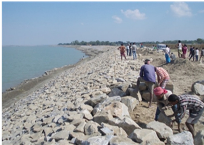
Figure 6: Use of boulder in bank revetment.
