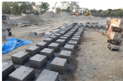
Figure 9: PCC blocks for bank revetment.
