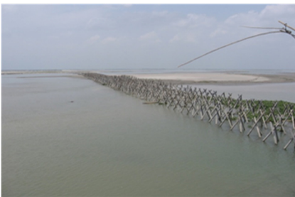
Figure 8: RCC porcupine for erosion protection.
