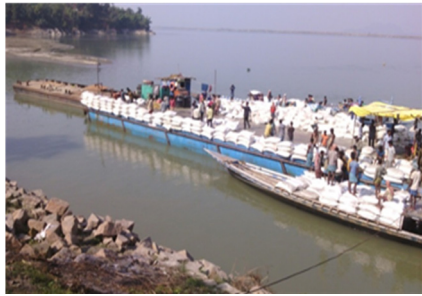
Figure 7: Dumping of geo bags near bank.
