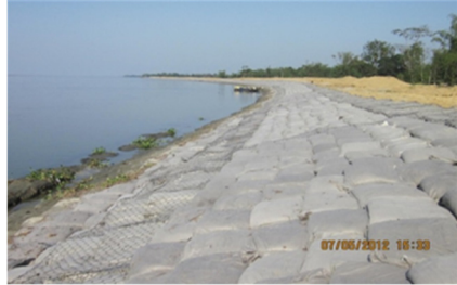
Figure 5: Geo synthetic bags in bank revetment.
