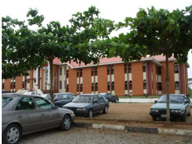
Figure 6: School of Earth and Mineral Sciences, Federal University of Technology, Akure. Use of brick facing as wall finishing
