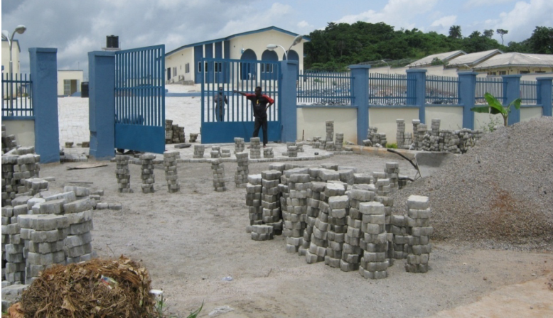
Figure 4: Unused interlocking tiles, granite and refuses on a recently completed building project.
