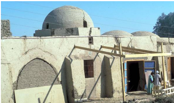
Figure 10: Adaptation of the original buildings of the village [4].
