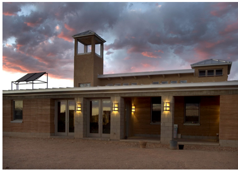
Figure 3: South facade of residence (photograph by Wilson Graham).
