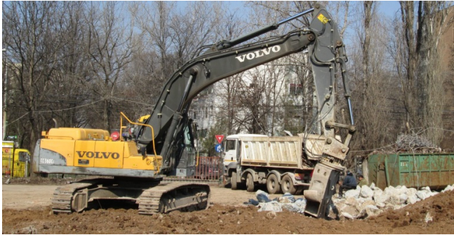
Figure 8: Demolition equipment on site.
