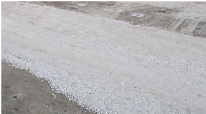
Figure 11: Filling with recycled aggregates.
