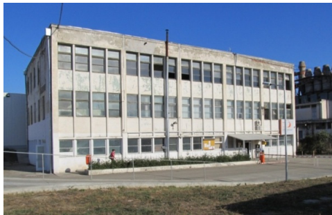
Figure 7: Multi-storey building to demolish.
