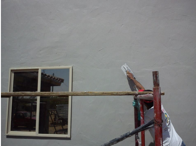
Figure 2: Paper plaster applied to a wheat straw wall.
