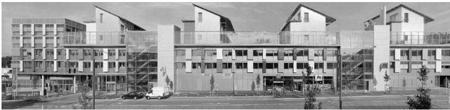
Figure 2: Sonnenschiff, plus-energy-houses, Architect Rolf Disch, Image: Th. Spiegelhalter.
