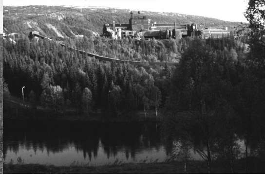
Figure 10: E and C Corneil. Steelworks and conveyor, Mo-i-Rana, Norway. Photograph 1990.
