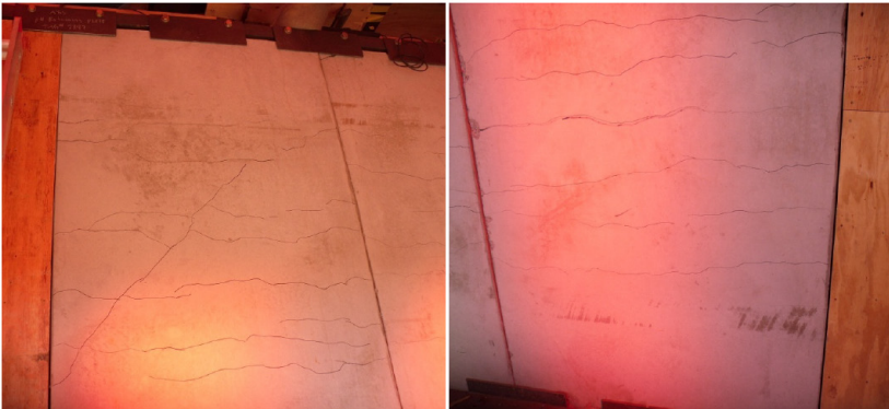
Figure 9: Post-test image of minor surface cracks in protected concrete panels.
