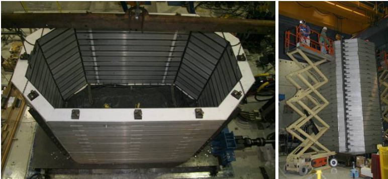
Figure 2: Assembly of laminar container at the University at Buffalo.
