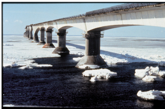
Figure 3: Confederation Bridge (Canada) while under construction (Bercha Group [11]).
