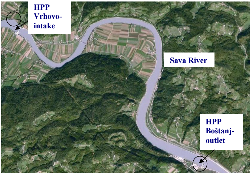
Figure 1: Reservoir of the HPP Boštanj.
