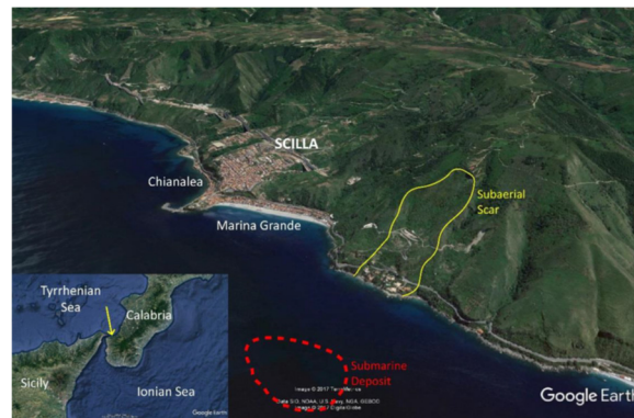
Figure 3: View of Scilla and its surroundings including the two main beaches of Marina Grande and Chianalea (see the position in the map in the bottom left corner). The yellow contour delimits the landslide scar (subaerial) measuring approximately 750\text{ m} \times 400\text{ m} , about 1 km west of the town. The red contour marks the submarine deposit observed in the geo-marine surveys [38]. (Source: Satellite view obtained by Google Earth [27].)
