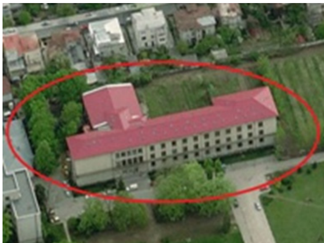
Figure 4: General view of faculty building.
