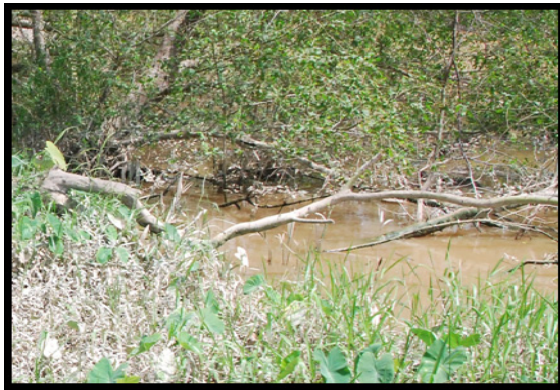
Figure 1: Typical sheet erosion along Langat River at Kuala Langat district.
