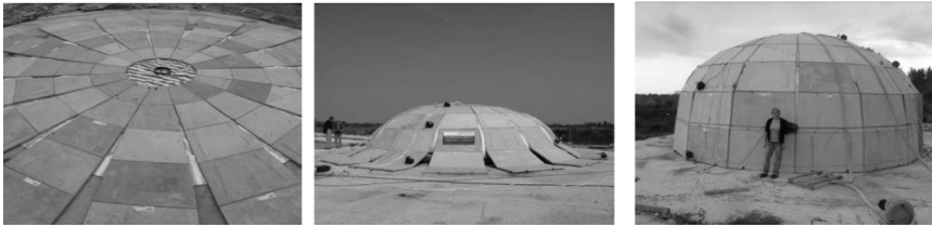
Figure 3: Pneumatic formwork for the erection of prefabricated concrete panels [10].
