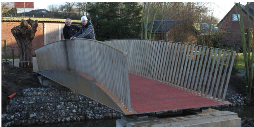
Figure 3: Designers G. Pauwels and N. De Temmerman standing on the lightweight curved bridge deck in corten steel (yet to become weathered).
