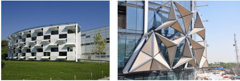
Figure 9: The Kiefer Technic Showroom located in Austria [17] (left); Picture showing the installation of the dynamic shading elements of the Abu Dhabi Investment Council [18] (right).
