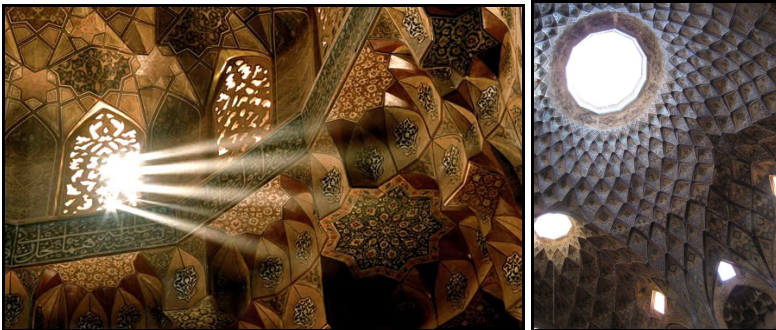
Figure 7: Light as a transformer. The Mugharnass under the dome reflect the light (left: Sheikh Lotfollah mosque), (right: Borujerdiha house).
