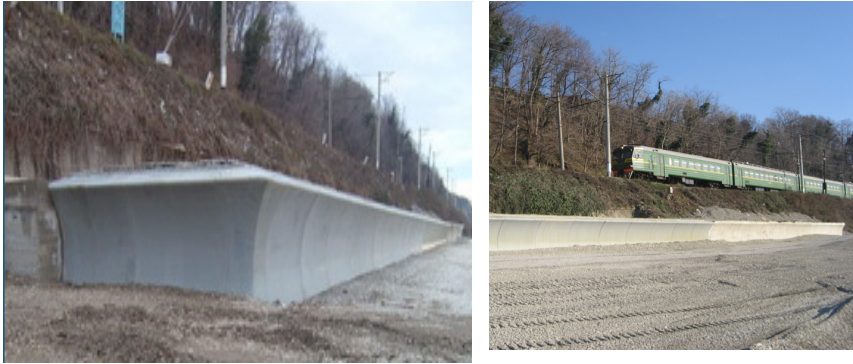
Figure 7: General overview of a composite material seawall.
