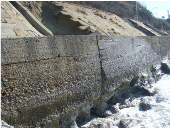
Figure 3: Reach-through slots in a concrete seawall.
