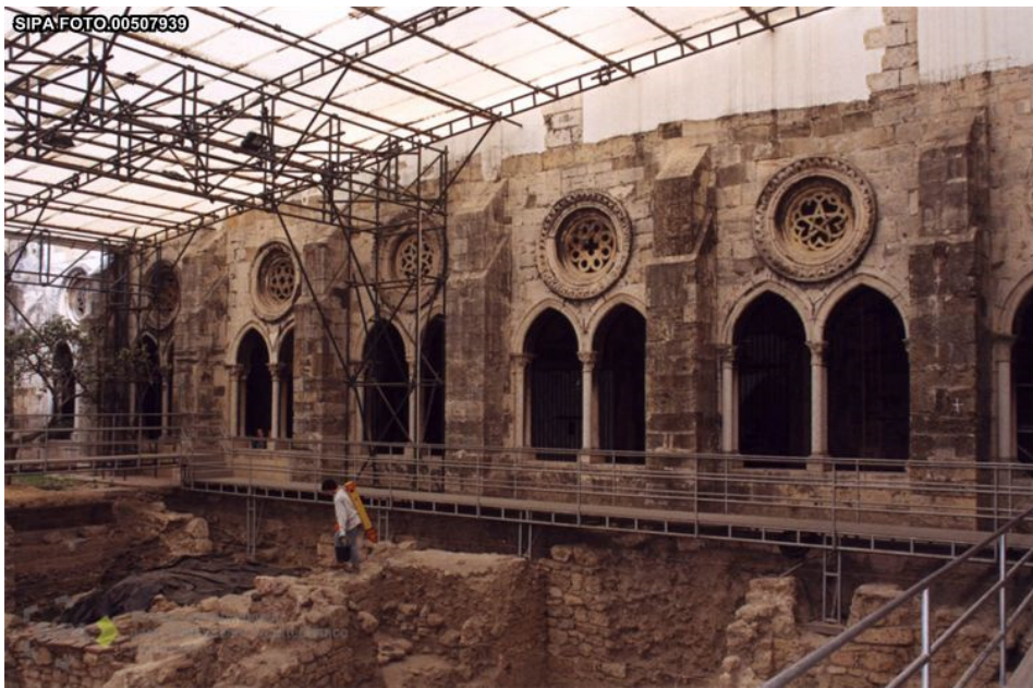
Figure 1: Excavations at the Lisbon cathedral.
