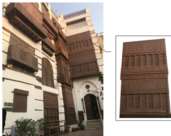
Figure 2: The Roshan in the Jeddah historic district.
