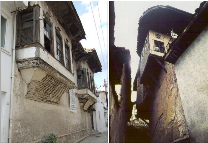
Figure 4: The blank façades at ground level, projections trying to make visual connection with the street and cages covering the windows for privacy, left one from Muğla, 2010. (Source: Güven Ulusoy, personal archive.) The right one from Bursa [10].
