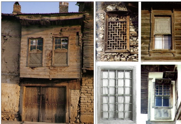
Figure 10: The privacy components of the house first floor: latticed windows with cages and different wooden crafts left from Isparta [9], right [11].
