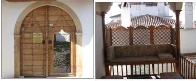
Figure 11: (a) The privacy components of the house: the kuzulu kapı of the Muğla house that enables entry of people and vehicles from different openings and strengthens privacy; (b) A sitting space in the sofa that enables people to perceive the street from cages by a projection. (Source: Güven Ulusoy personal archive.)
