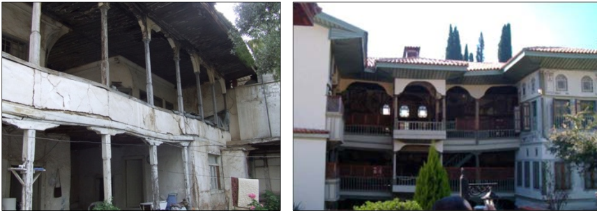
Figure 7: Photos showing the semi-open spaces called aiwan and hayat/sofa . Left is from Muğla (2010), right from Birgi Çakırağa Mansion (2008). (Source: Güven Ulusoy personal archive.)
