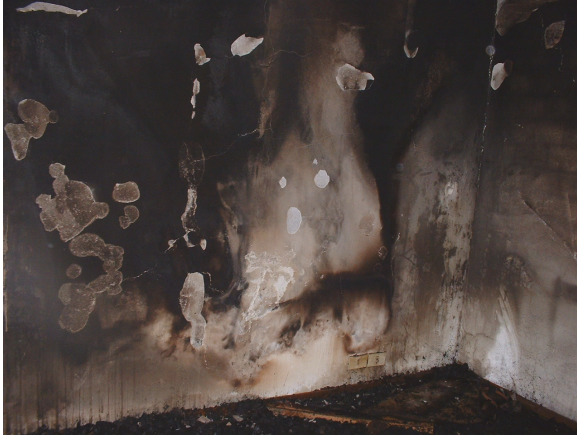
Figure 4: Detail of one wall in the room originating the fire. The wardrobe gone completely destroyed was located near this wall.
