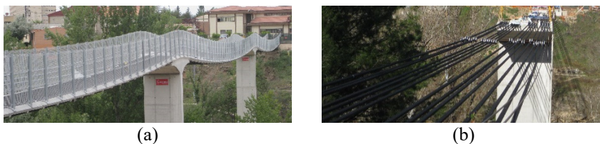
Figure 1: Views of the stress ribbon footbridge. (a) Overall view; and (b) Detail of carbon fiber cables.
