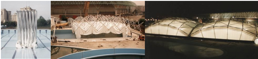
Figure 1: Deployable cover for swimming pool in Seville designed by Escrig and Sanchez [7].
