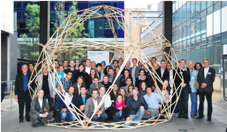
Figure 1: A transformable scissor structure dome based on the principle of the USC (Universal Scissor Component). Built at Imperial College in September 2011 during the SMG (Structural Morphology Group) International Seminar.
