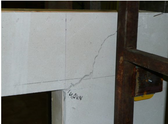
Figure 8: The appearance of the first crack in the O3 test samples.
