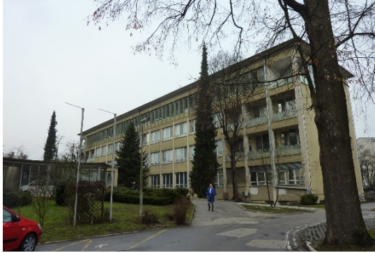
Figure 7: Case study hospital building.
